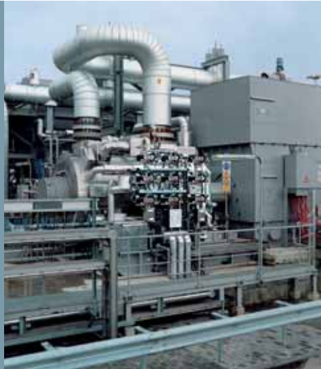
23-MW motor running at 6,300 rpm to pump gas south of Groningen/The Netherlands
